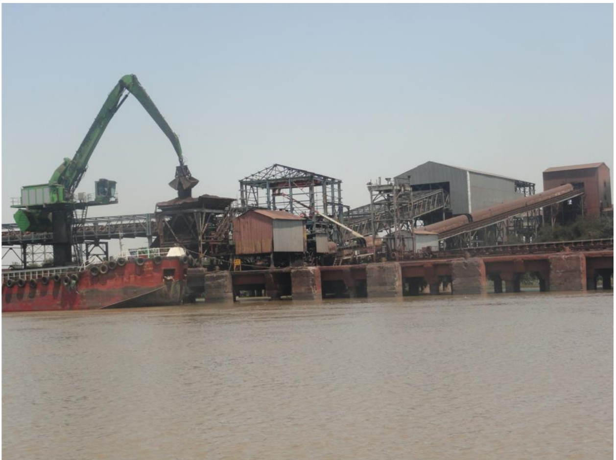
Figure 15: Picture showing crane and conveyor belt in operation at Dharamtar port.
